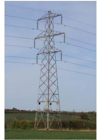
132kV DC lattice
